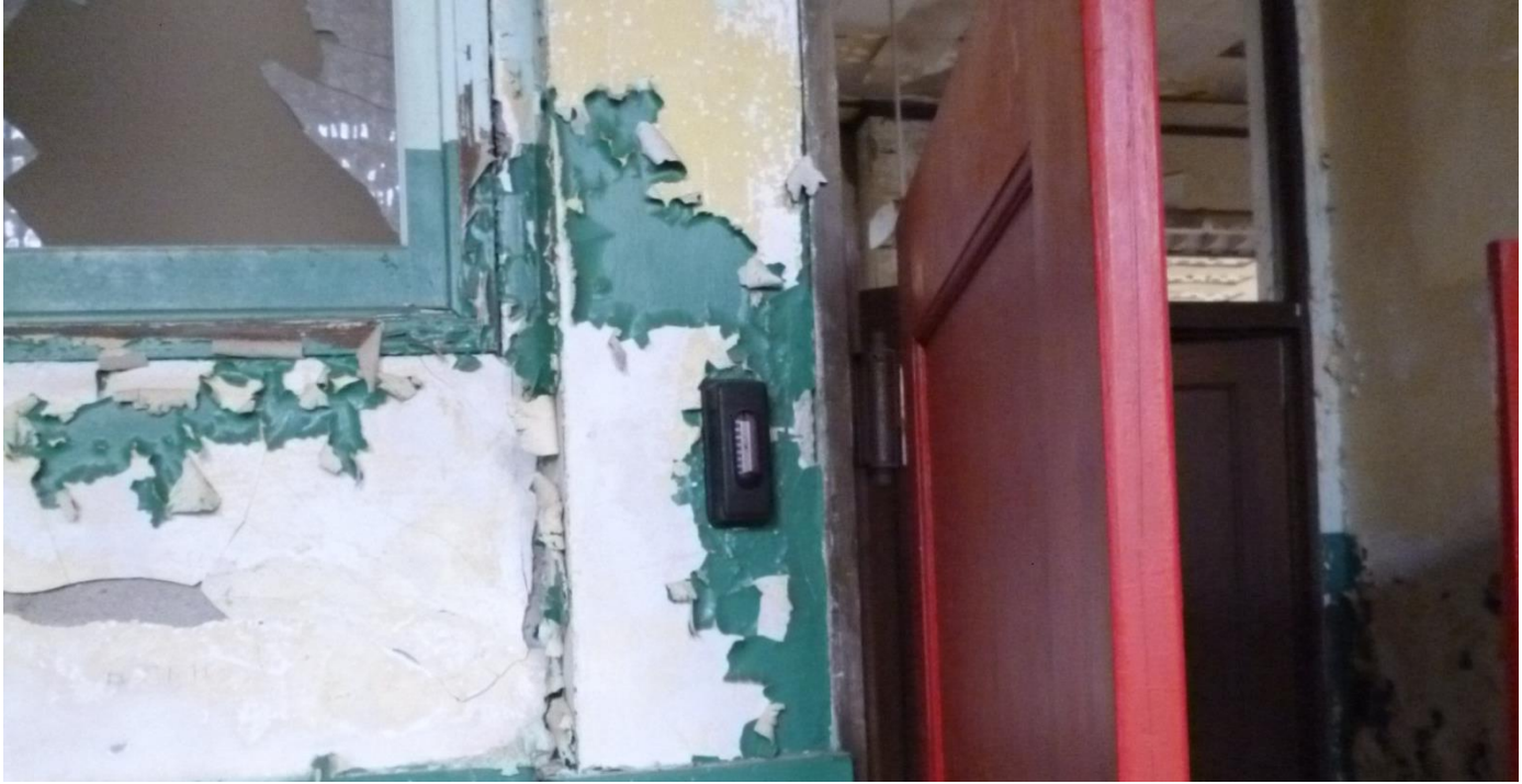
Chipping lead-based paint observed during a basement water sample analysis at the former Silver Creek Elementary / High school, 60 Main Street Silver Creek, NY.
